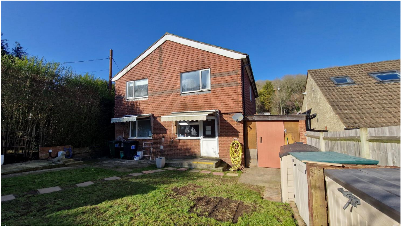
Figure 7: Photo of Rear Elevation
